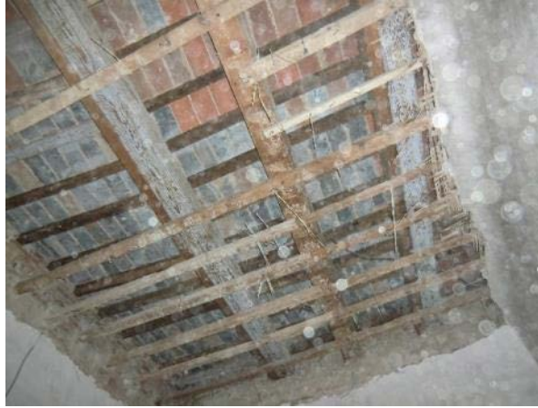
Solai in putrelle e tavelloni
